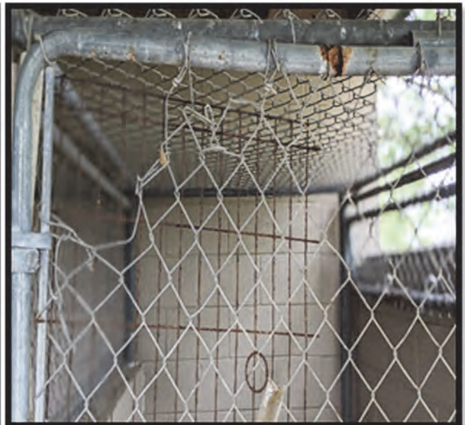
Deteriorating, corroded existing kennels.
