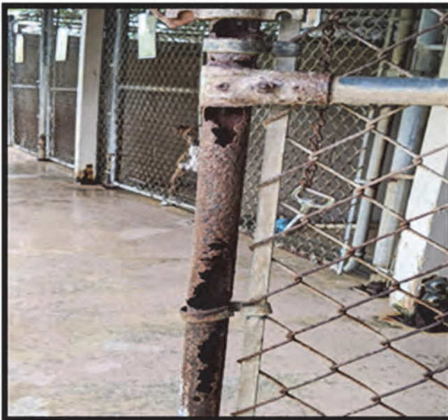
Deteriorating, corroded existing kennels.
